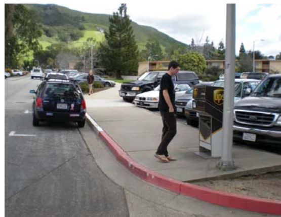
Figure 9.1.C: There are many obstructions that prevent the correct implementation of a curb ramp.
