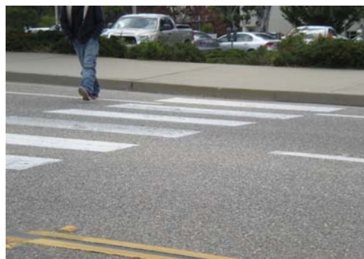
Figure 9.2.B: The crosswalk has a curb ramp on the side not shown.
