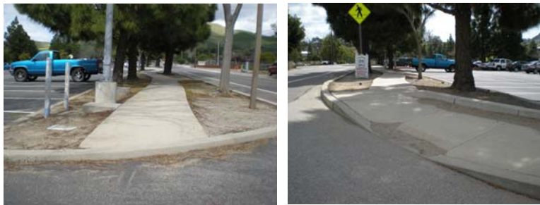
Figure 9.1.E: The sidewalk has a curb ramp leading up on to it but not off.
