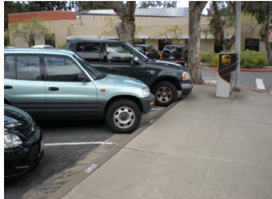
Figure 9.1.B: Although a person can get to this point in a wheelchair, there is no way for the person to get down off the sidewalk.
