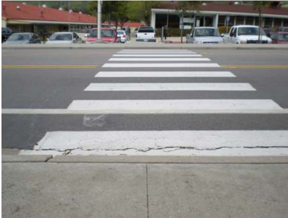
Figure 9.2.A: The crosswalk does not have curb ramps on either side.
