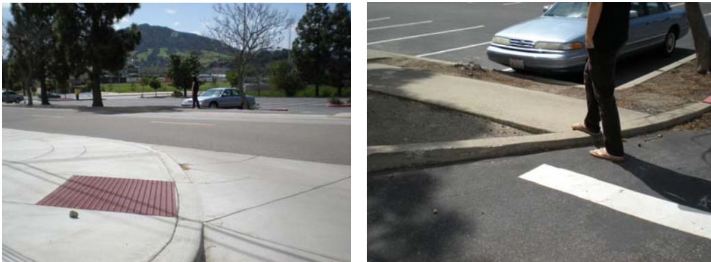
Figure 9.1.D: The sidewalk on the other sidewalk lacks a corresponding curb ramp.
