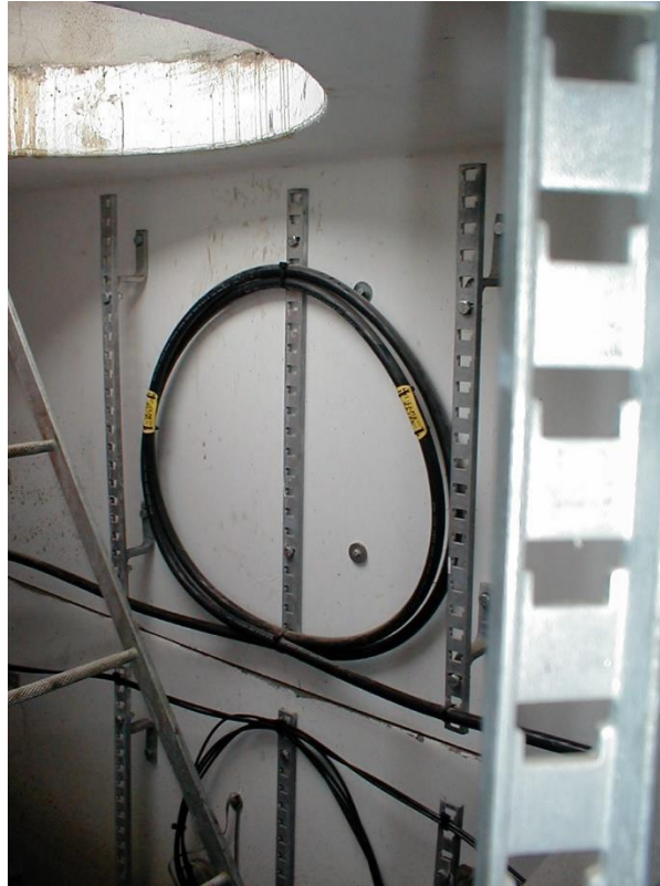
Exhibit 1 - Fiber Service Loop in a Manhole
