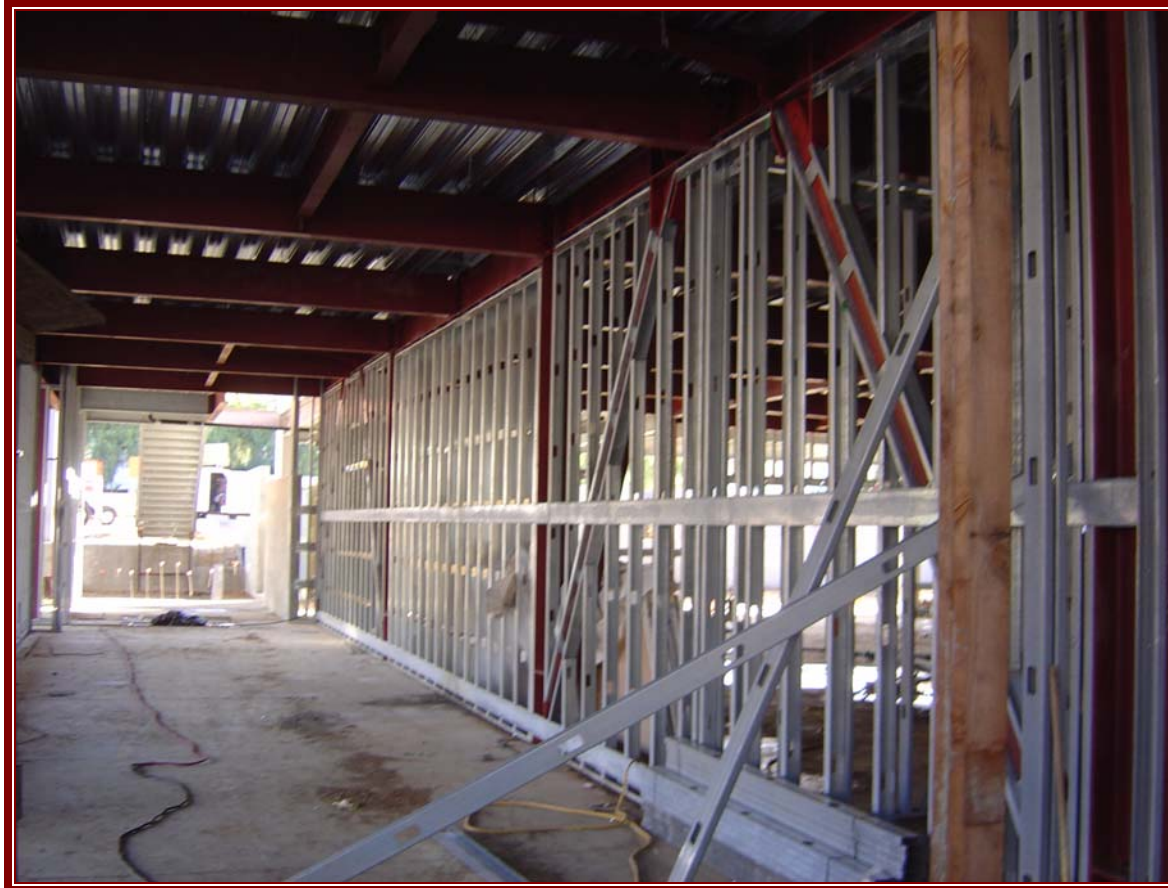
Cal Poly SLO - Bonderson Projects Center – View of Interior Wall In-fill for the exterior and interior walls is created by the use of metal studs manufactured from recycled steel.
