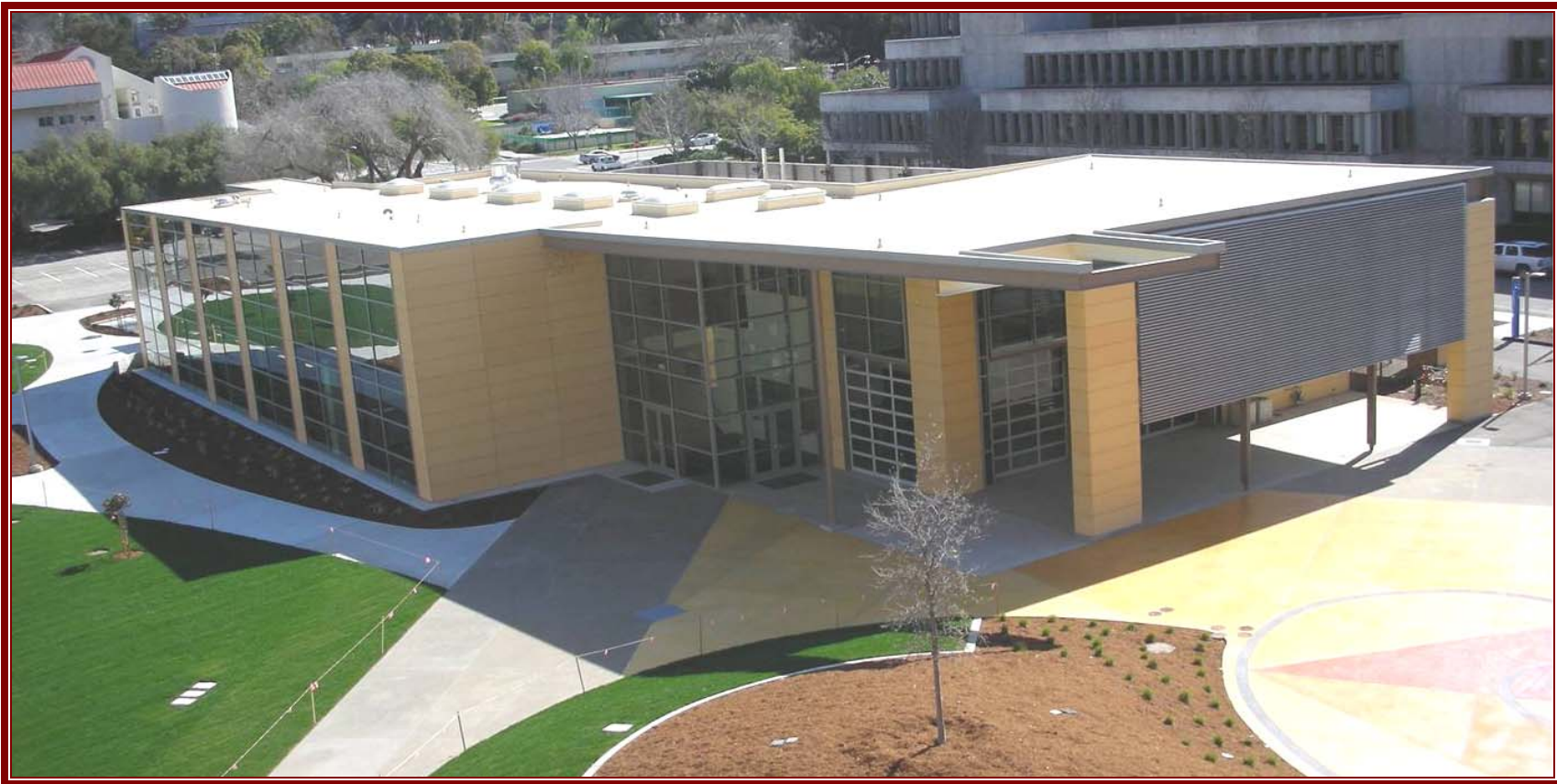
Cal Poly SLO - Bonderson Projects Center - View from North Glazing on the west side of the building provides daylighting to the west entrance and the Project Integration work room. A deep overhang and louvers shade the glass in the afternoon, while still allowing daylight into the building. The deep overhang also provides protection for an outdoor display area.
