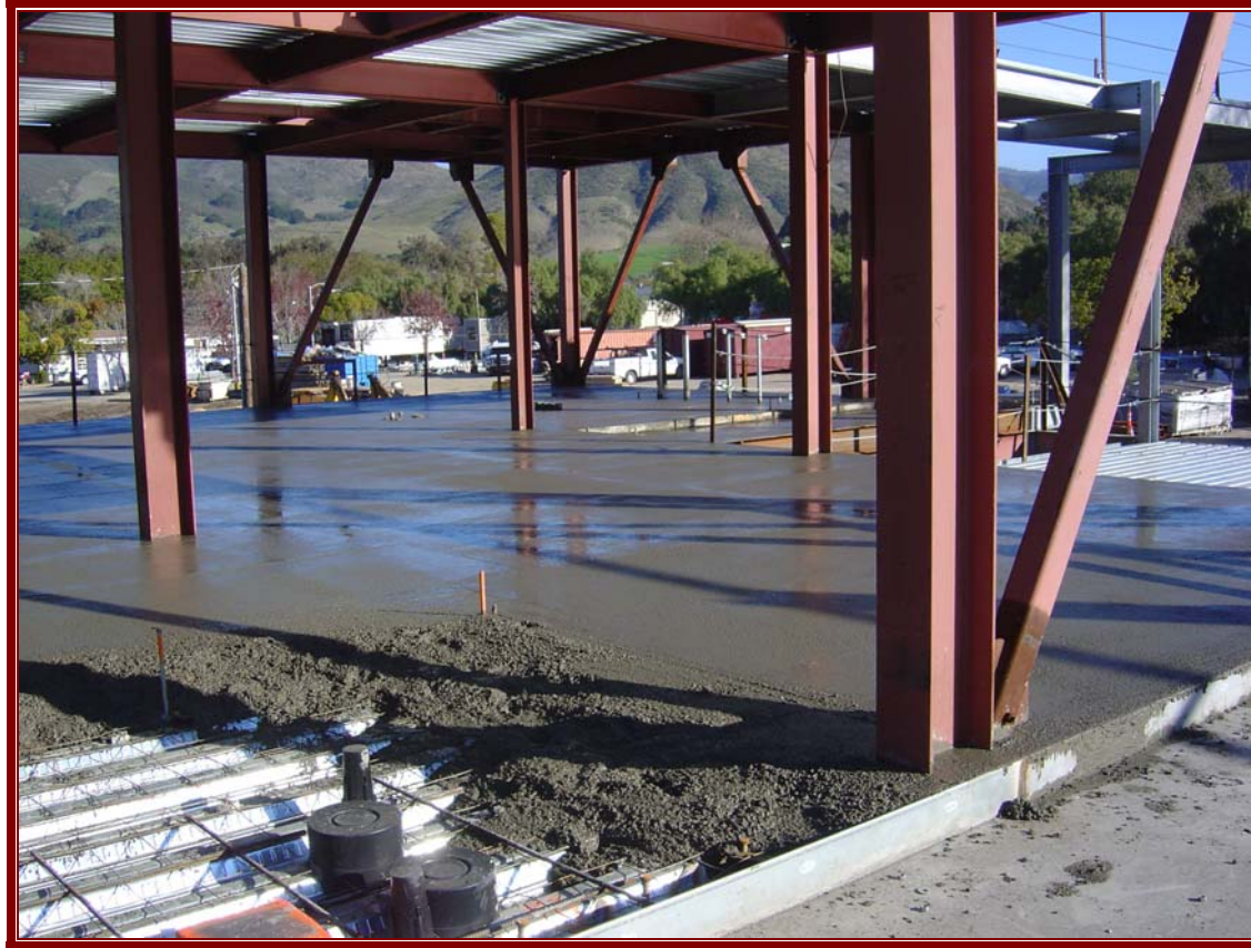
Cal Poly SLO - Bonderson Projects Center – View of Structural Steel The structural system is made from recycled steel and includes rebar used in the concrete slabs, columns, beams and corrugated metal decking.
