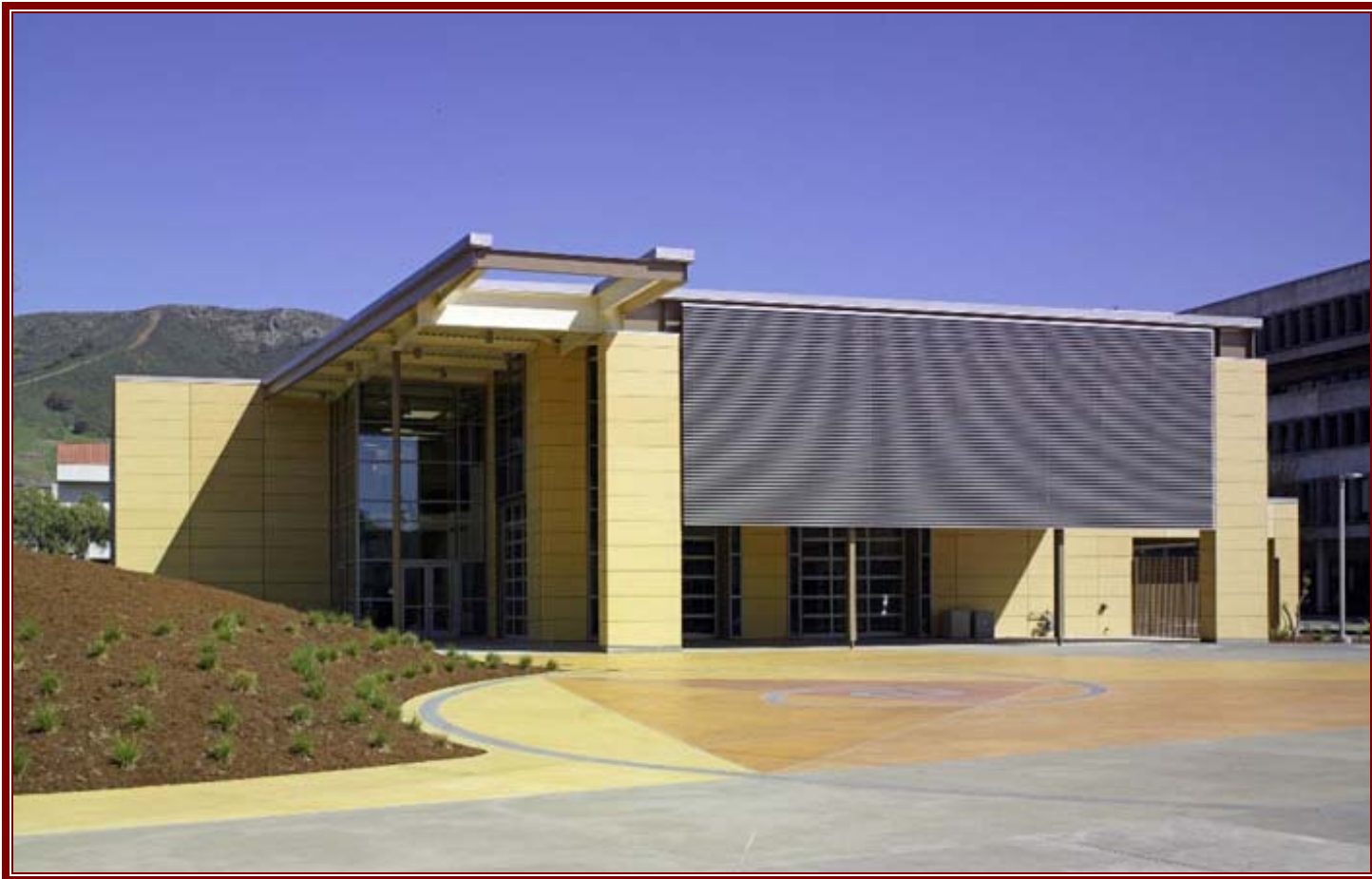
Cal Poly SLO - Bonderson Projects Center – View from West The glazing at the west entrance and the Project Integration work room is shaded from the afternoon sun by deep overhangs and louvers.
