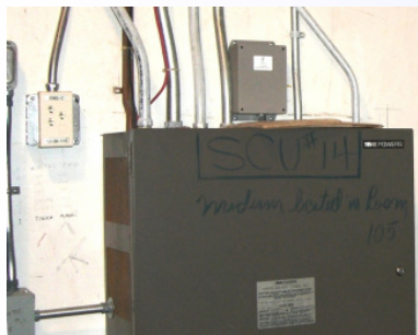
Web-to-Wireless Gateway (WWG) transmits sensor data to Federspiel Supervisory Controller (FSC)
