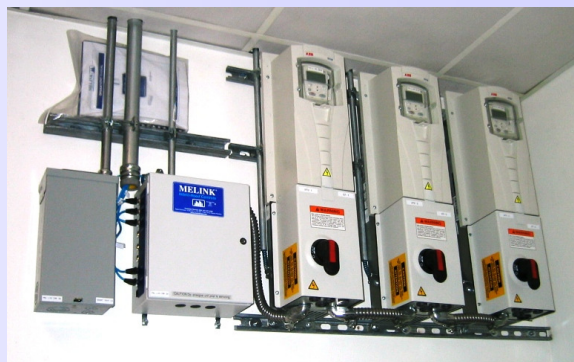
Melink processor panel and fan motor VFDs
