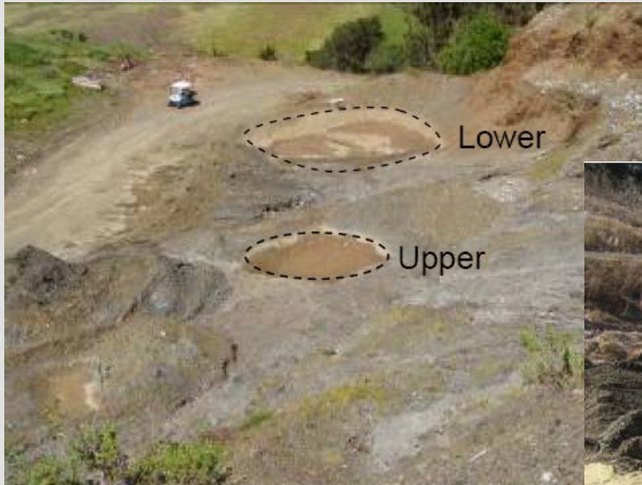
Figure 23: Overview of detention basins Apr 05
