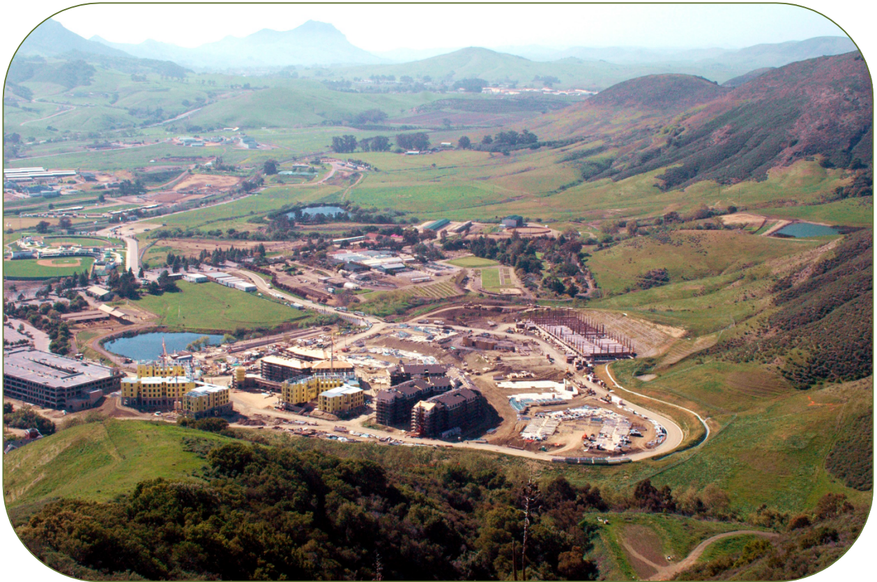
Photo: Poly Canyon Village construction by Kevin Waldron
