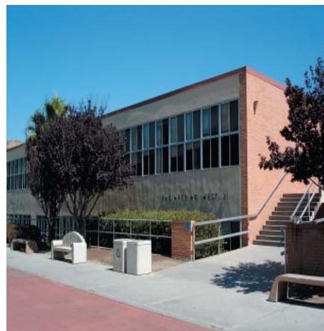
One of only three CSU campuses to take advantage of a systemwide program, Cal Poly installed photovoltaic panels on Engineering West in 2006.
