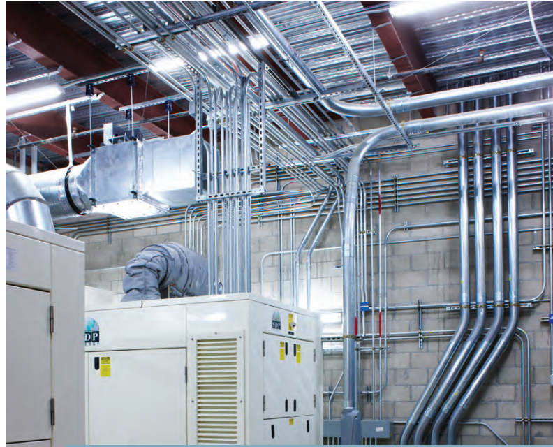
PCV Co-generation. Poly Canyon Village uses a co-generation process: the waste heat from two high efficiency on-site electricity generators provides space heating and domestic hot water for the complex, as well as heating the swimming pool.
